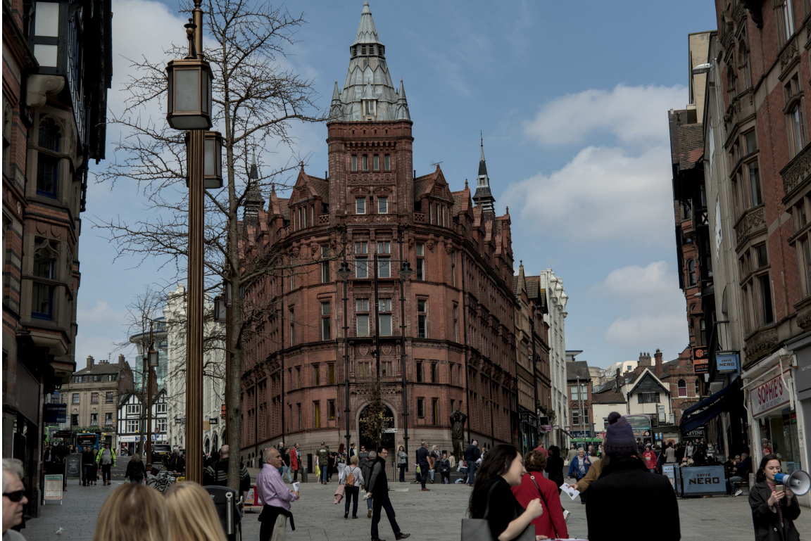
F47A4583 - Prudential Assurance Building.
