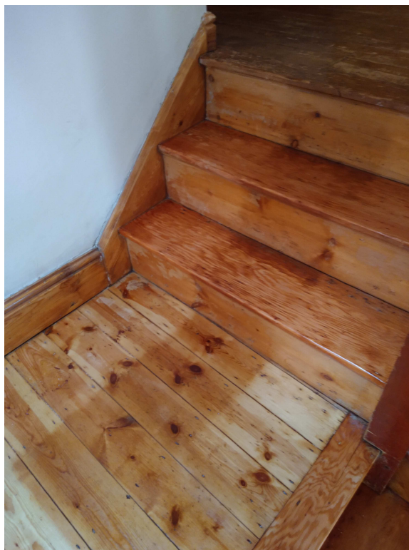
IMG_081740107 - The stairs.
