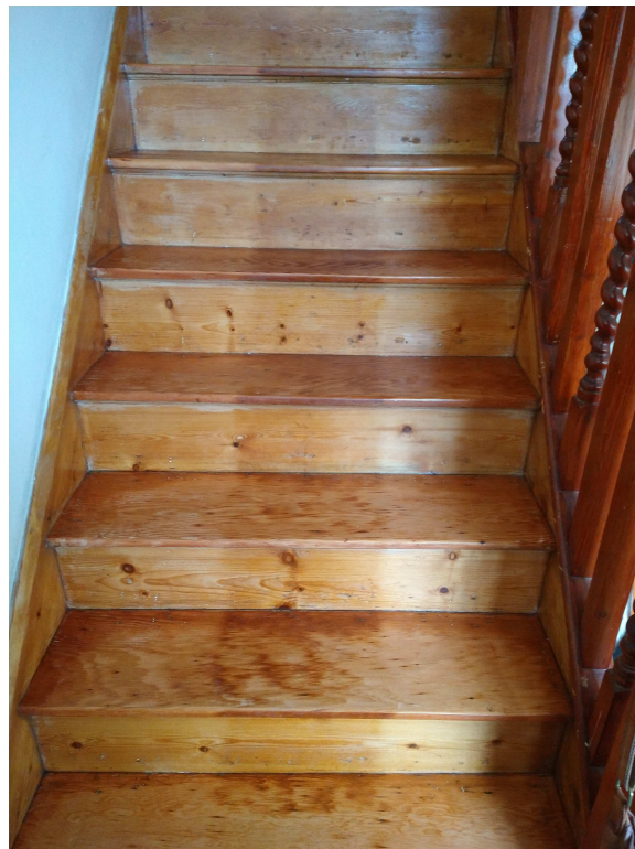
IMG_081702317 - The stairs.
