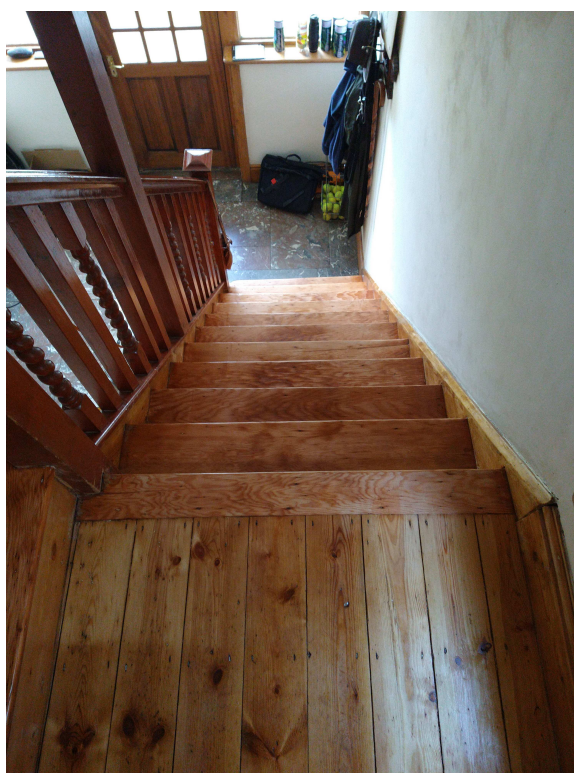
IMG_081754792 - The stairs.
