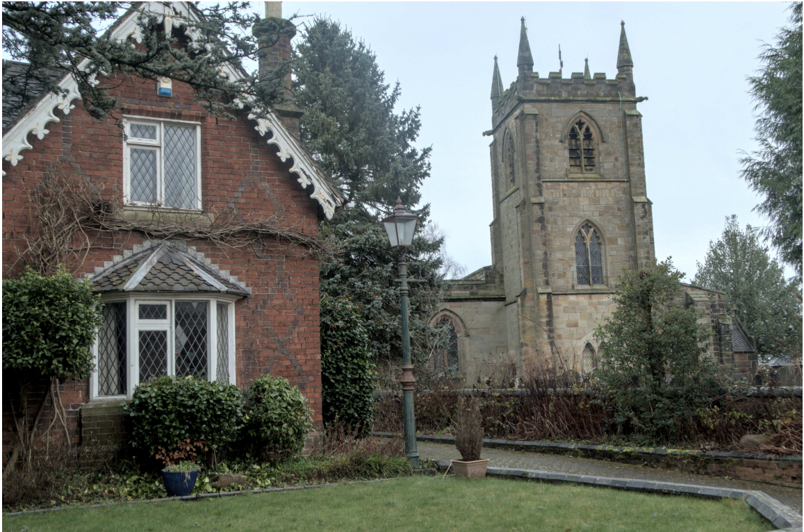
P1035986 - House and church tower.
