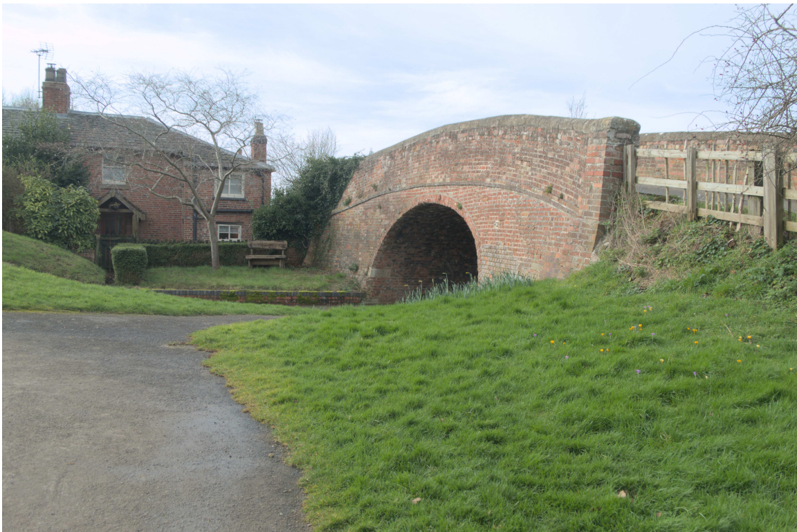
P1036089 - Bridge and cottage.
