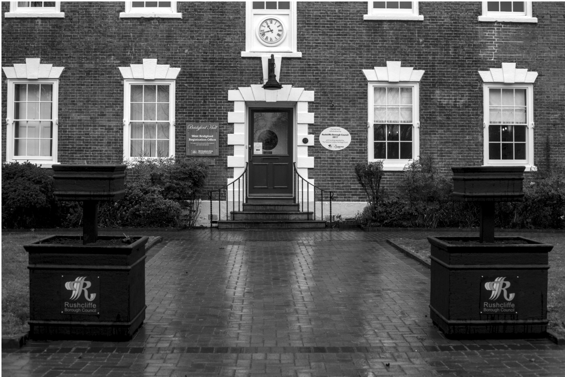
F47B6341 - Bridgford Hall after rain.
