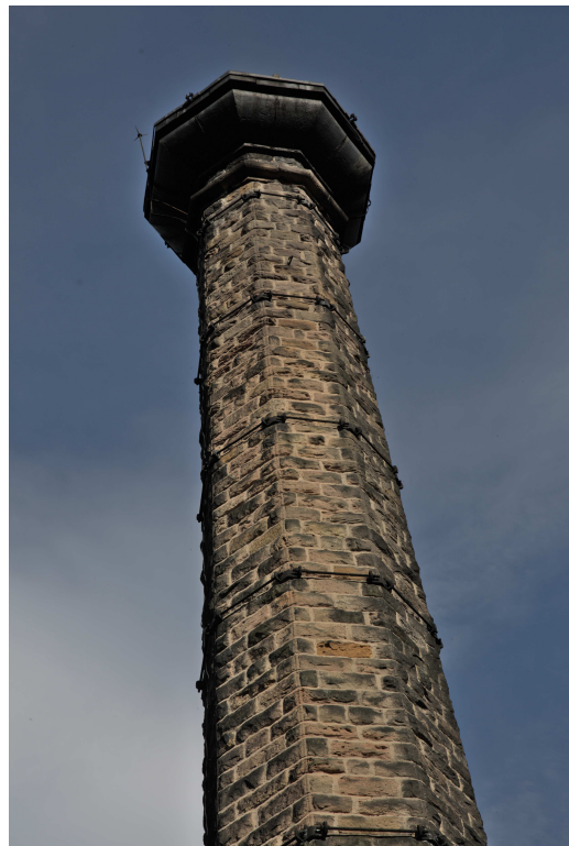
F47B7526 - Chimney stack.
