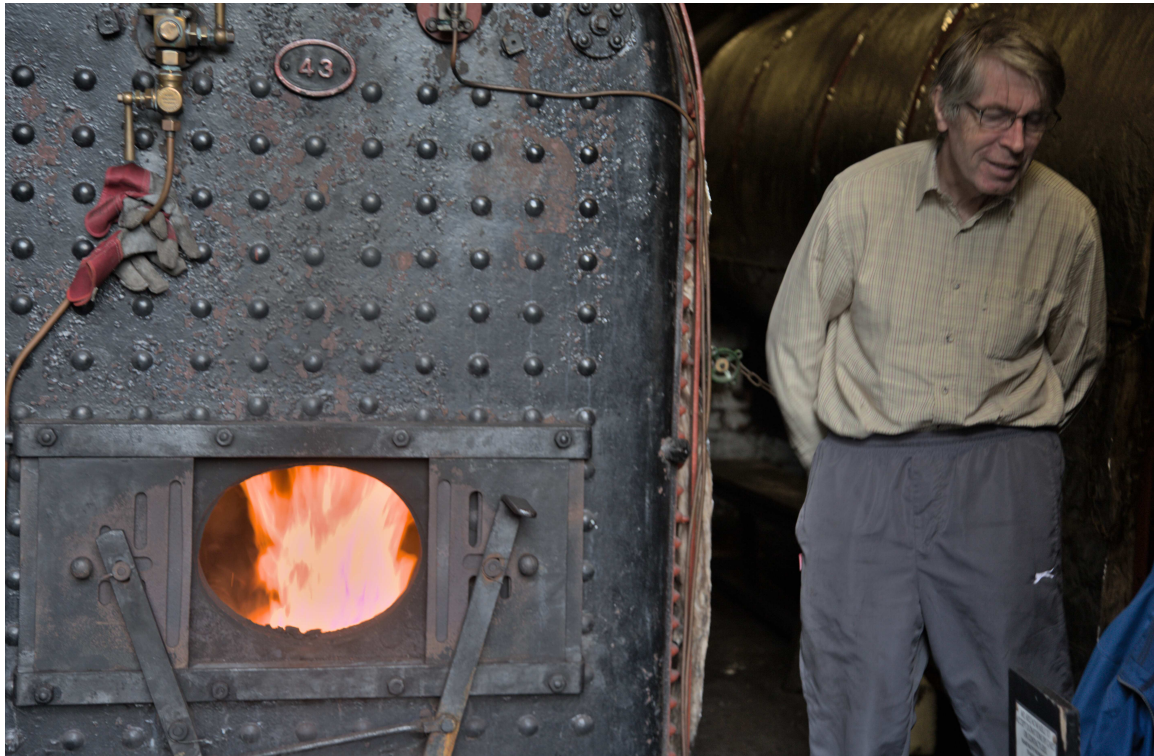
F47B7524 - Midland Railway locomotive boiler.
