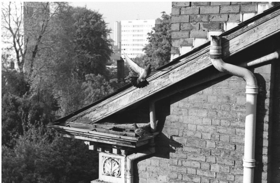
ZO4-A0021 - Eaves Gough Road.
