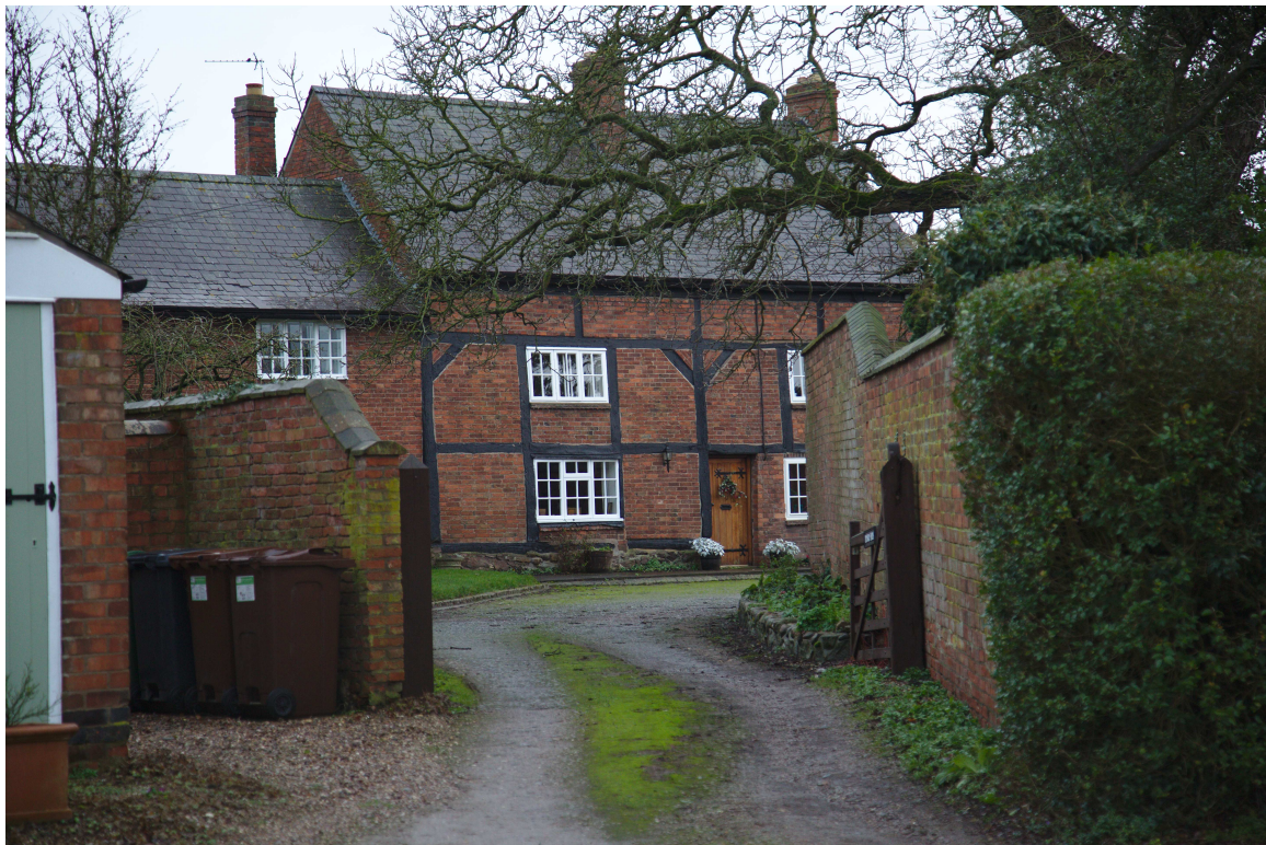
Wood framed brick built house.
