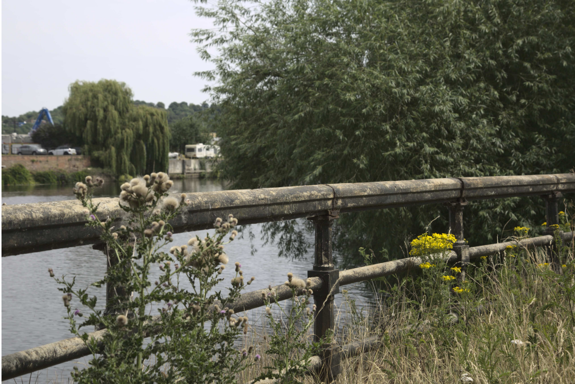
F47B5157 - Old riverside railing.
