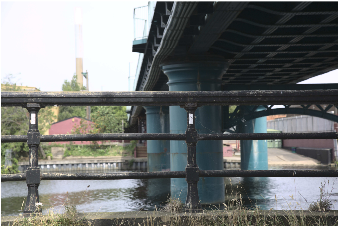
F47B5155 - Lady Bay Bridge.
